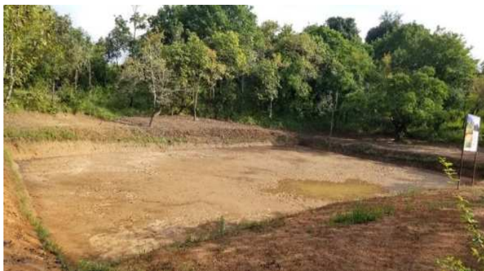
Figure 3: Constructed water recharge pond, Darma Rural Municipality
